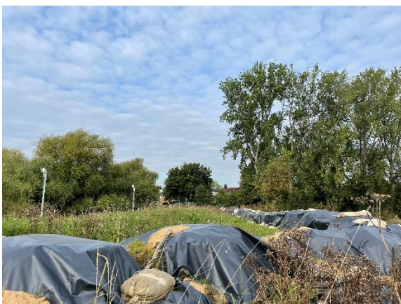
Current temporary repairs along the bank at Wheel Hall Farm
